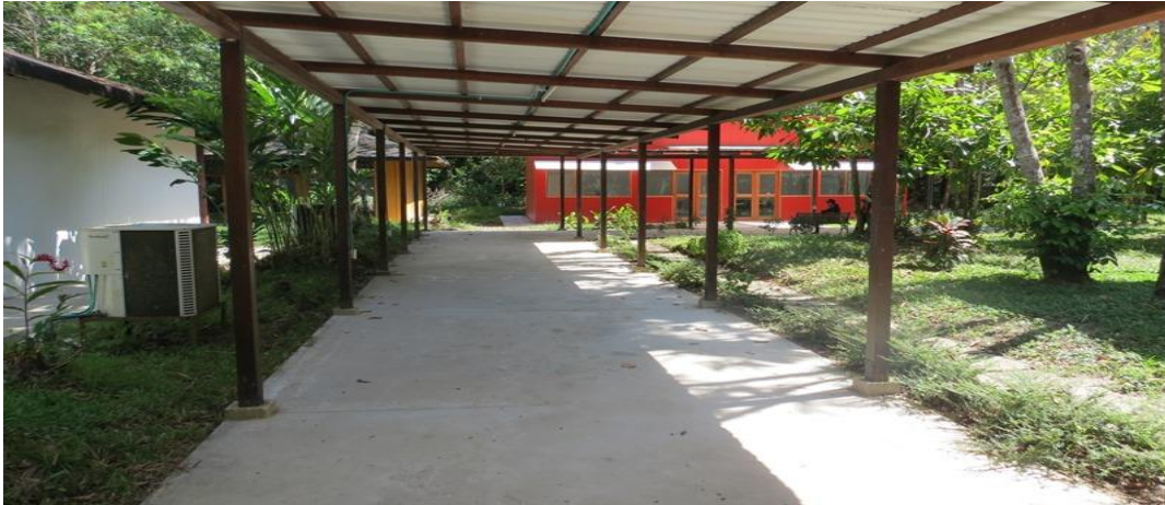
Foto 3. Aulas TIC. Sept 2015
